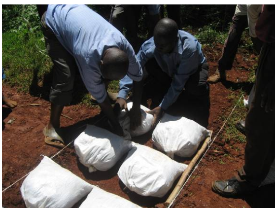
Figure 10. “Do-nou” are positioned at a site where the mud has been removed. The space between “Do-nou” is necessary to allow them to expand due to compaction (Kenya)
