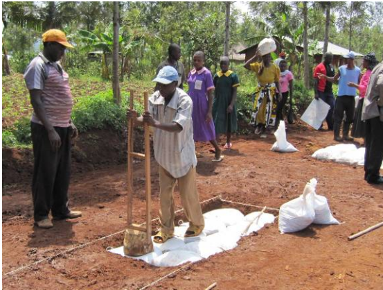
Figure 11. A villager is compacting “Do-nou” using a wooden mallet (Kenya)
