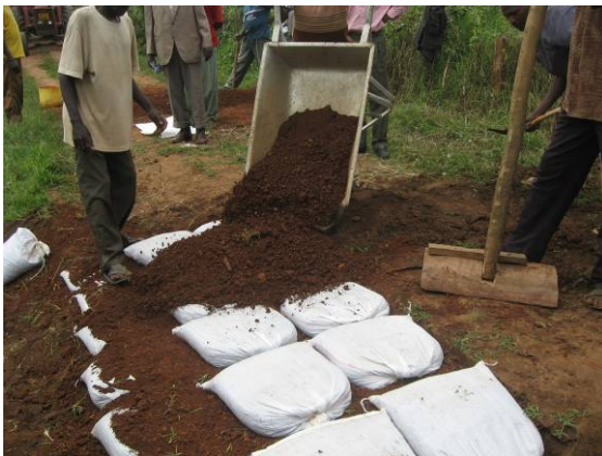
Figure 12. Gravel is distributed over the final layer of “Do-nou” to build the layer of the road surface (Kenya)
